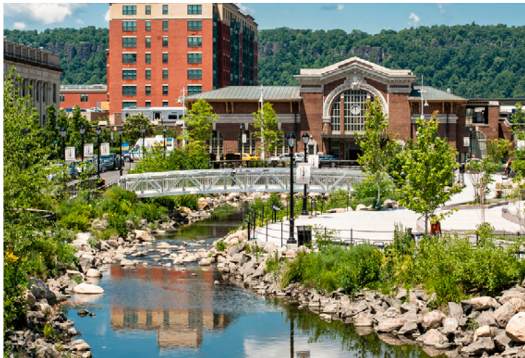
Saw Mill River Daylighting Project Yonkers, NY
