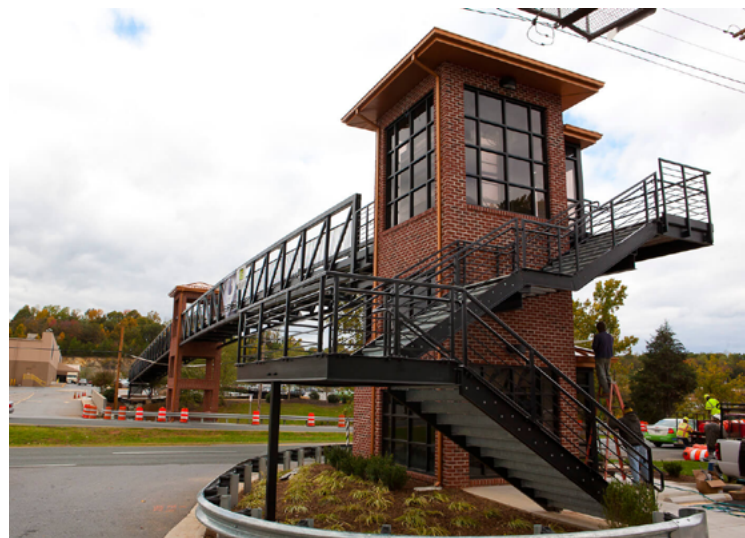
Wards Road Pedestrian Bridge Lynchburg, VA
