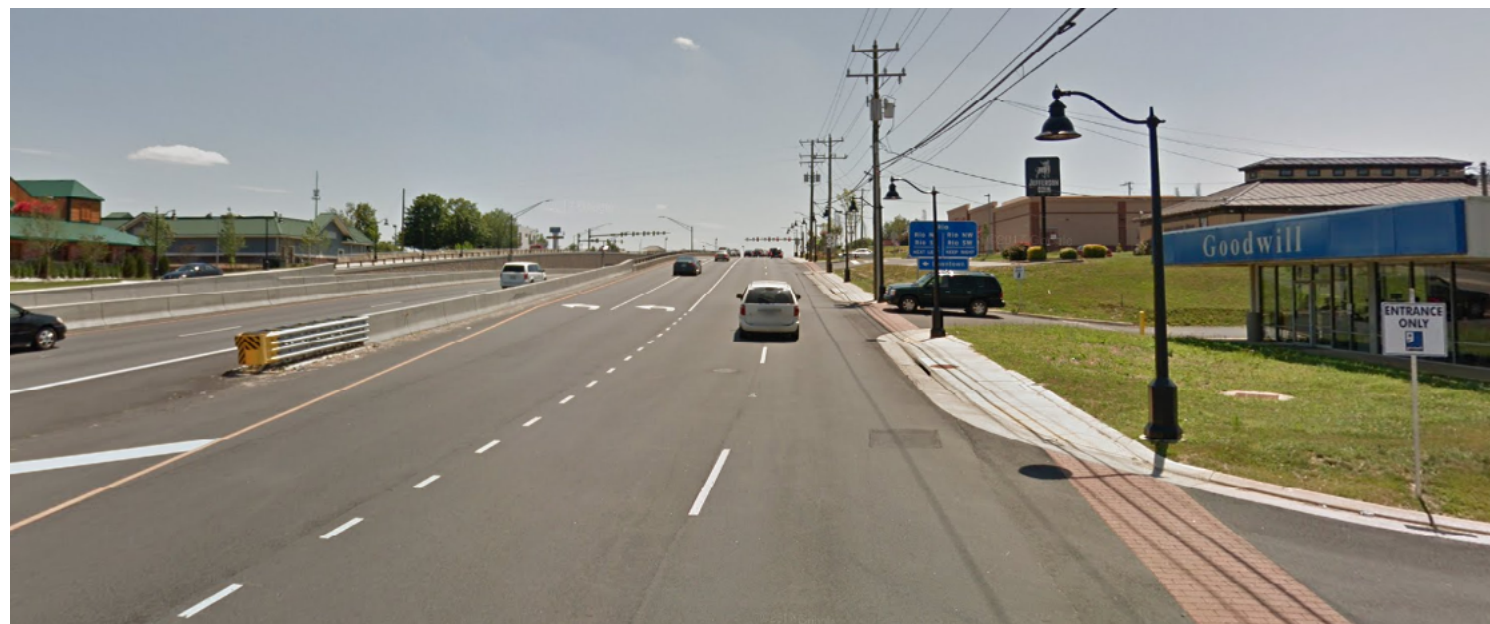
Existing Conditions: Route 29 South on Ramp Approaching Rio Road
