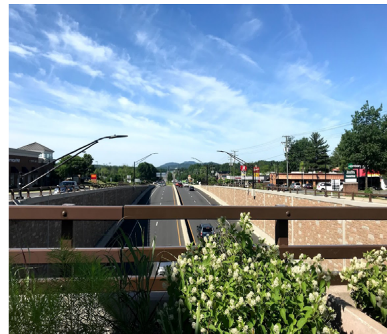
View from Rio29 GSI Looking South
