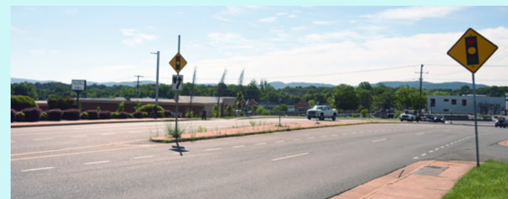
Rio Road West, Looking NE
