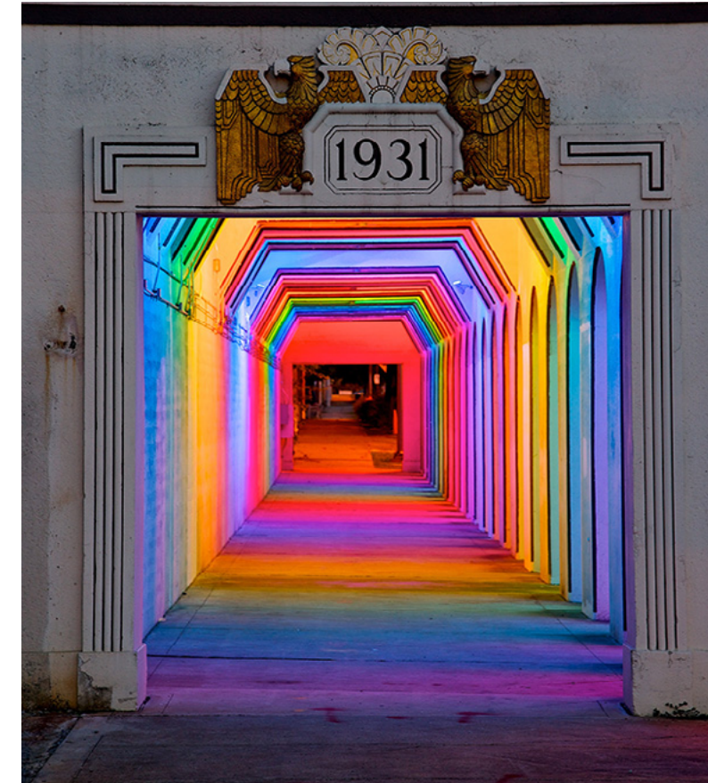
LightRails Pedestrian Underpass Birmingham, AL
