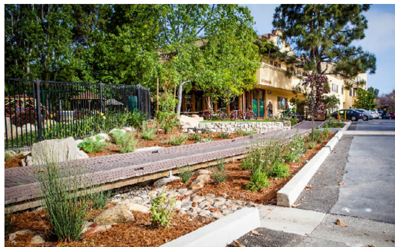
Bioswales Outside of a Shopping Center Ventura, CA
