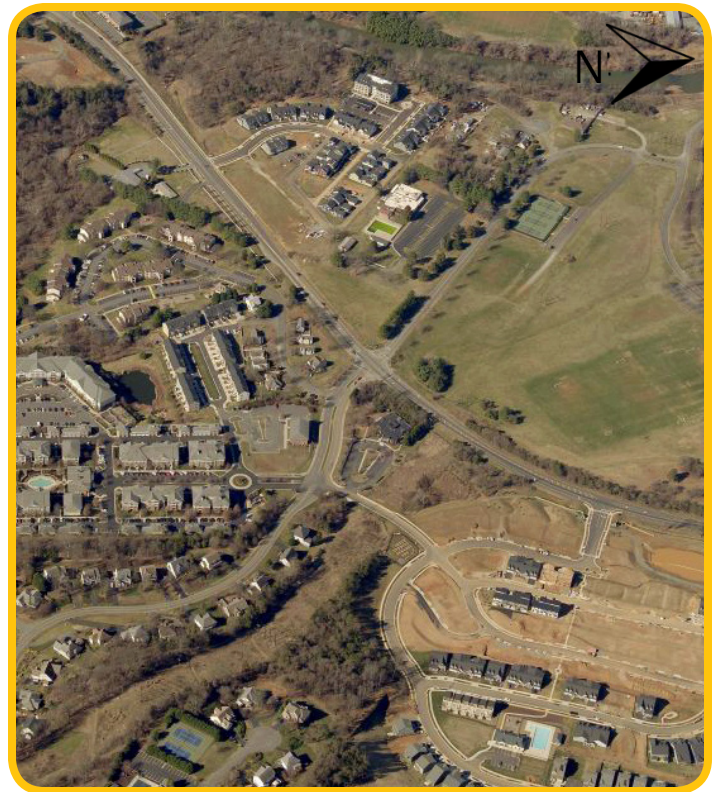
Neighborhood Service Center at the intersection of Elk Drive and Stony Point Road, facing southwest. Darden Towe Park can be seen in the upper right corner.
