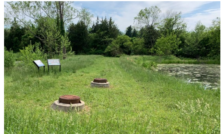
Stormwater management regulations provide requirements to treat runoff areas and capture sedimentation. Shown: stormwater management facility in Crozet.
