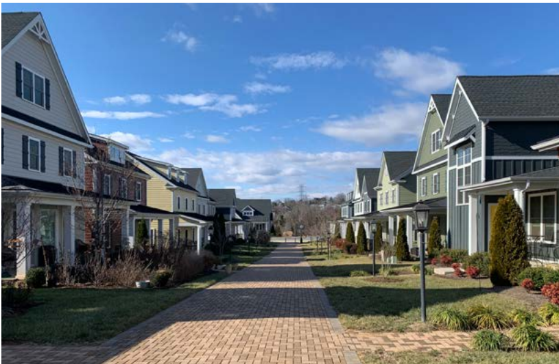
Cottage-style homes fronting a walkway with garage access in the rear.
