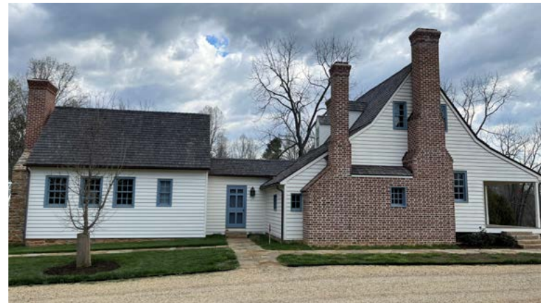
Images before and after the renovation of Findowrie, a historic farmhouse in the Southwest Mountains National Register Rural Historic District.
