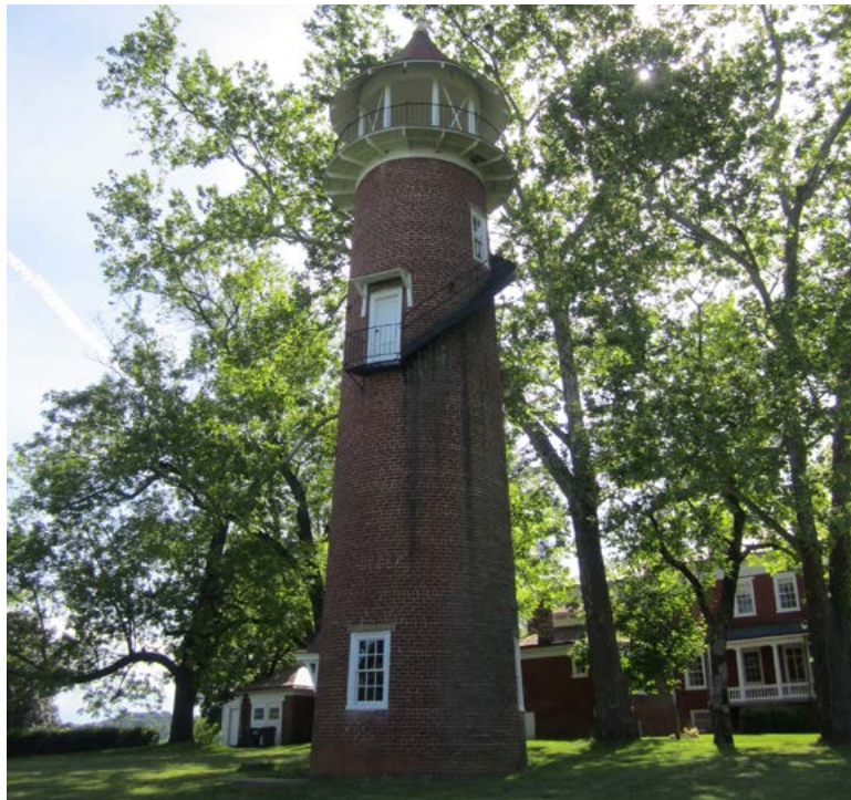
Historic water tower, Birdwood Mansion property.
