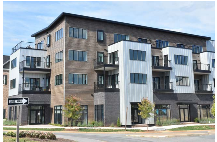
Multi-family developments help achieve recommended densities in the Development Areas. Top: parking lot awning with solar panels in the Riverbend neighborhood. Bottom: Old Trail apartments.
