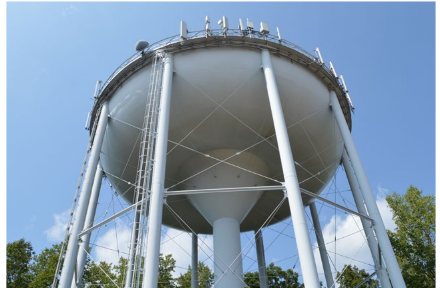
Water storage tower on Woodburn Road.
