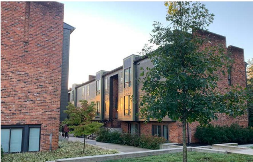
Park Lane Apartments have been renovated to improve energy efficiency.
