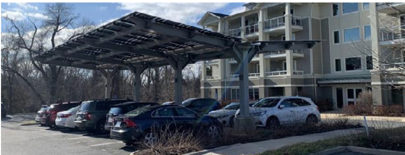
Parking lot awning with solar panels in the Riverbend neighborhood.
