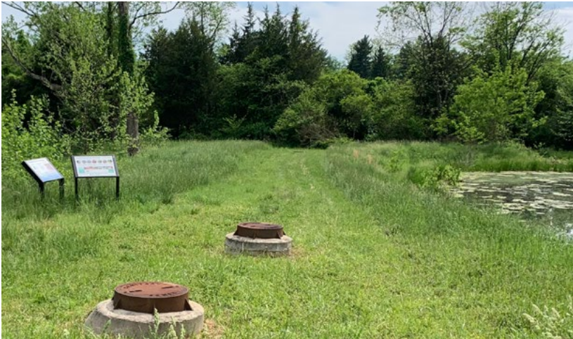
Stormwater management facility in Crozet.
