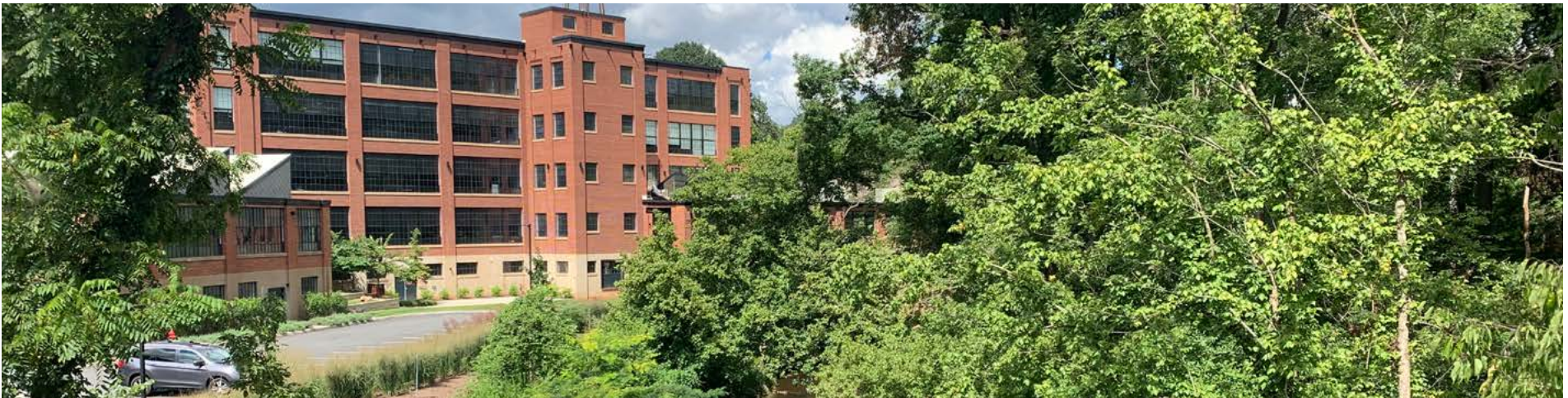
The Woolen Mills project renovated an existing industrial property and converted it to mixed use.
