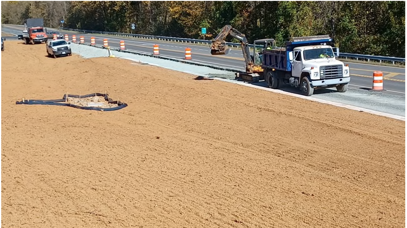
Biscuit Run Park Phase 1a paving prep work along Rt. 20
