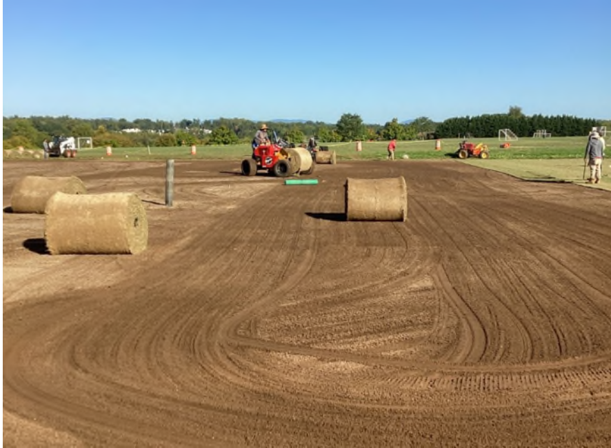
Sod being installed at Darden Towe Park
