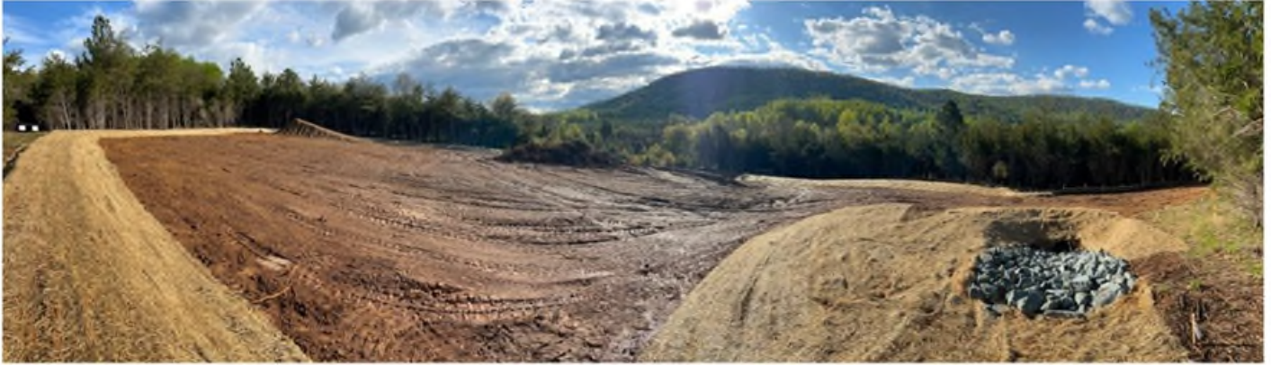
Grading and erosion control.
