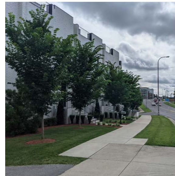
A large transition zone with enhanced plantings reinforces a residential character within an urban context
