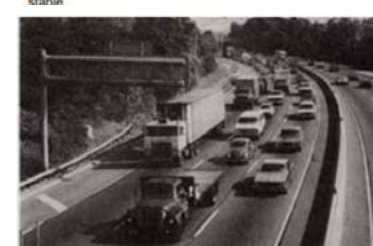
Level of Service E: Unstable flow at or near capacity levels with poor levels of comfort and convenience.
