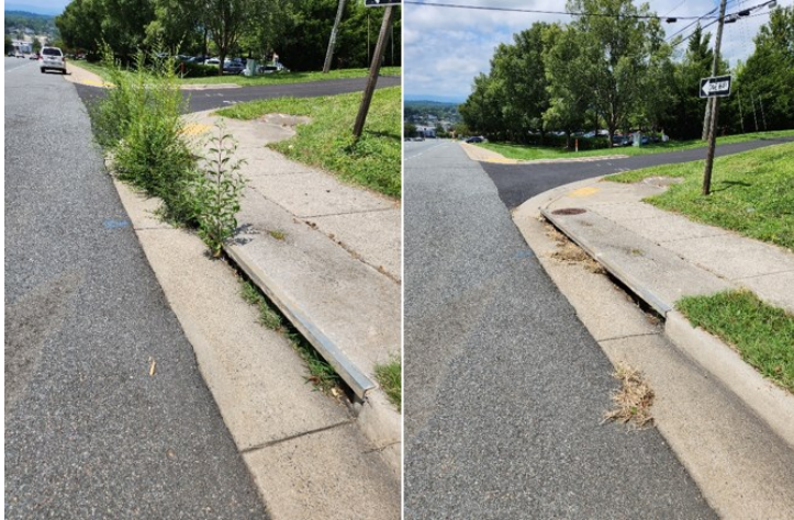
Pantops storm sewer curb inlet:
