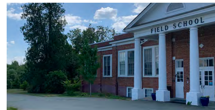
(above) An existing field on the site, looking toward the stream, and the Old Crozet School building.
