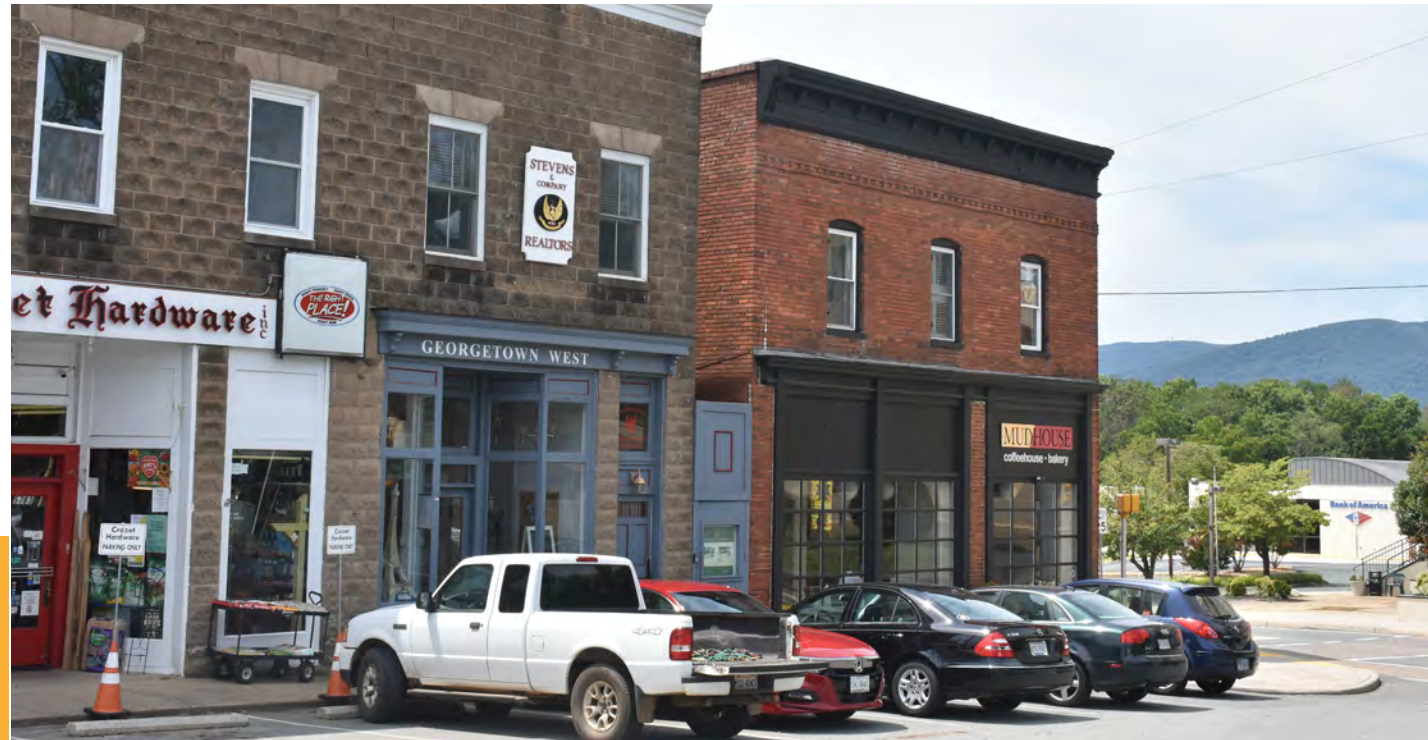
(above) The Square in Downtown Crozet is an iconic, focal point of the community, with a variety of retail, service and office uses.
